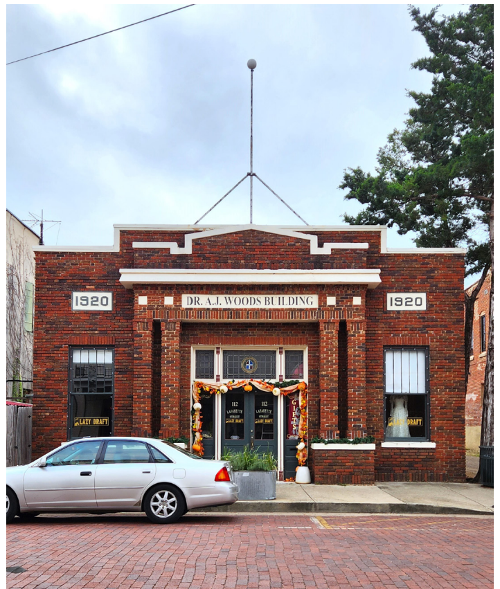
Figure 4.3: Dr. A.J. Woods Building (Source: Keerti Rath)
