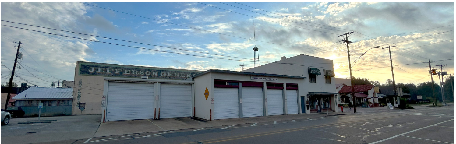
Figure 5.4: Jefferson Volunteer Fire Station (Source: Elizabeth Dupont)
